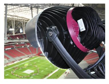
Figure 3. Large Die Cast Heat Sinks for High Power LED Stadium Lights [3]
